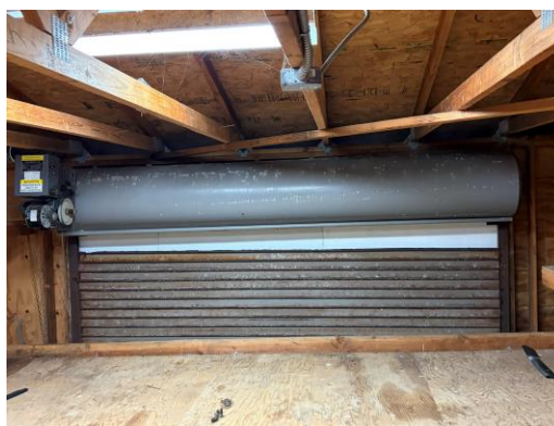
Figure 45: Coast Guard Building – Roll up door with door torn off from the top motor.
