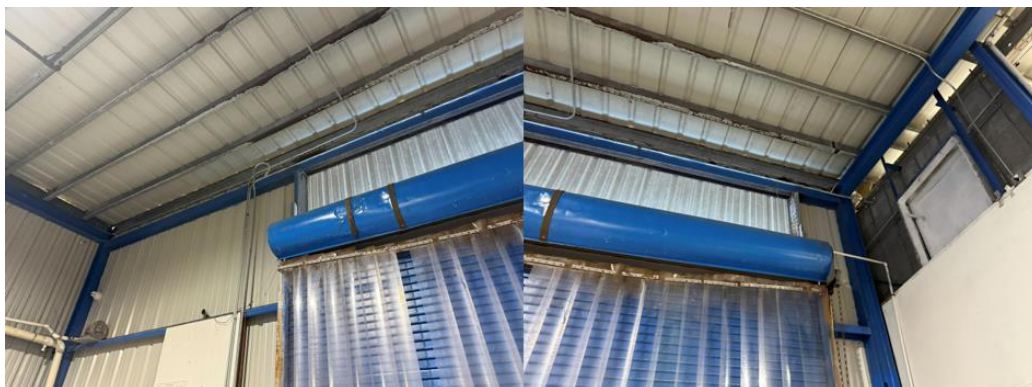
Figure 24: Fish Processing Facility 1 – North wall with roll up door.
