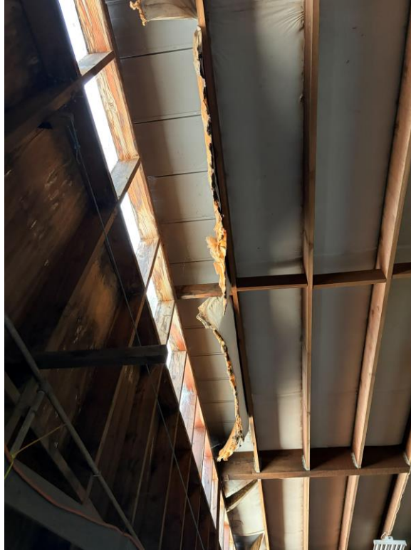
Figure 14: Boat Yard – Low Bay roof system, standing seam metal roof over wood rafters.
