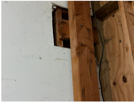
Figure 42: Coast Guard Building – Corner post frame to double wide mobile structure.
