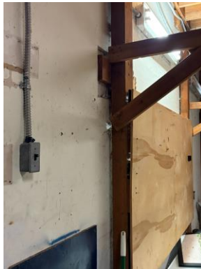
Figure 43: Coast Guard Building – Middle post frame to double wide mobile structure.
