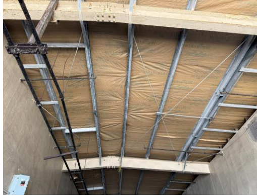
Figure 33: Fish Processing 2 – Roof cross bracing.
