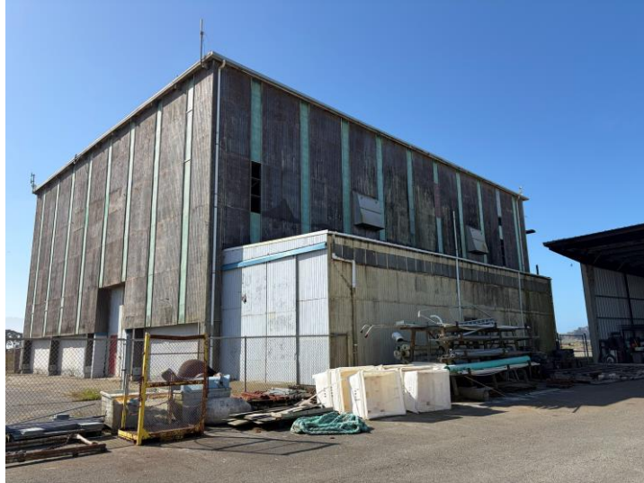
Figure 9: Boat Yard – Exterior siding for high and low bay.
