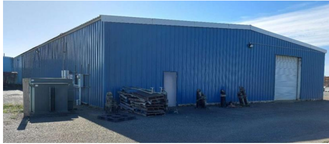
Figure 27: Fish Processing Facility 2 – Exterior of building.
