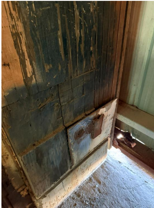
Figure 8: Boat Yard – Interior modified post at southeast corner.
