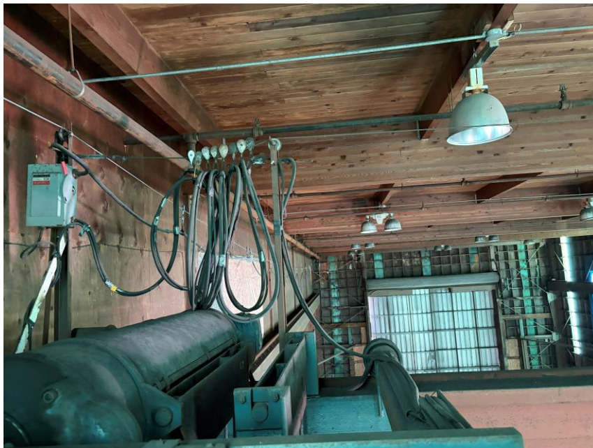
Figure 11: Boat Yard – Crane beam.
