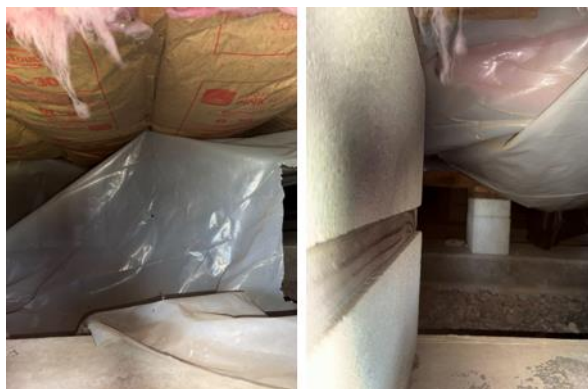
Figure 46: Coast Guard Building - Portable structural crawl space.
