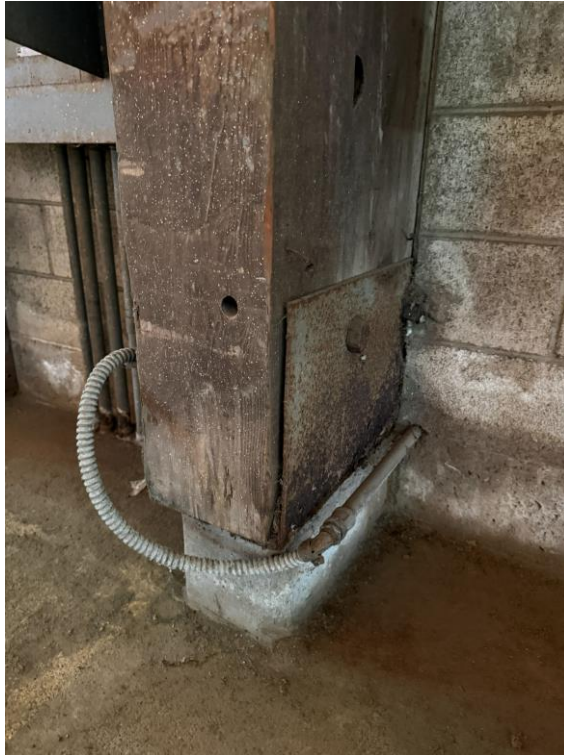
Figure 7: Boat Yard – Interior column with no visible damage
