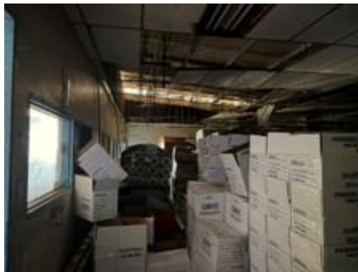
Figure 32: Fish Processing 2 – Interior space with miscellaneous materials.
