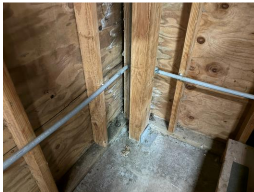
Figure 41: Coast Guard Building – Post foundation connection.
