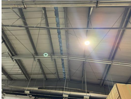
Figure 21: Fish Processing Facility 1 – Roof lateral cross bracing in original structure.
