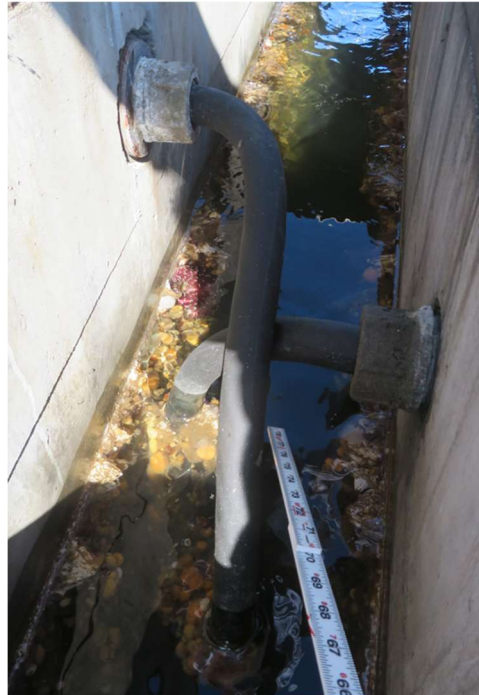
d) Wiring at HM09 to 10
