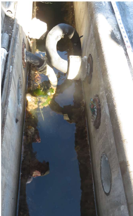
c) Wiring at HM05 to 06
